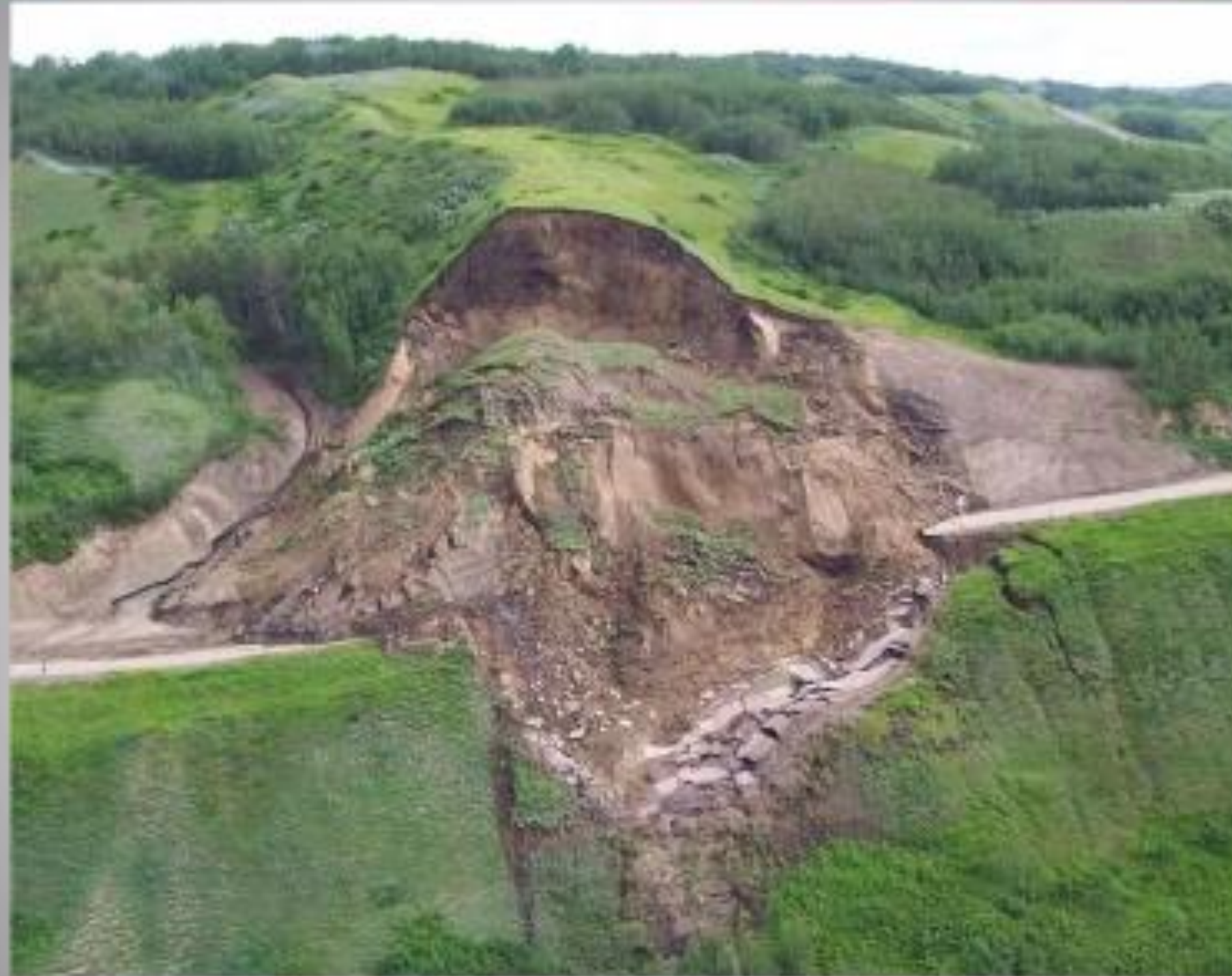
Fig. - Landslides or slip erosion
